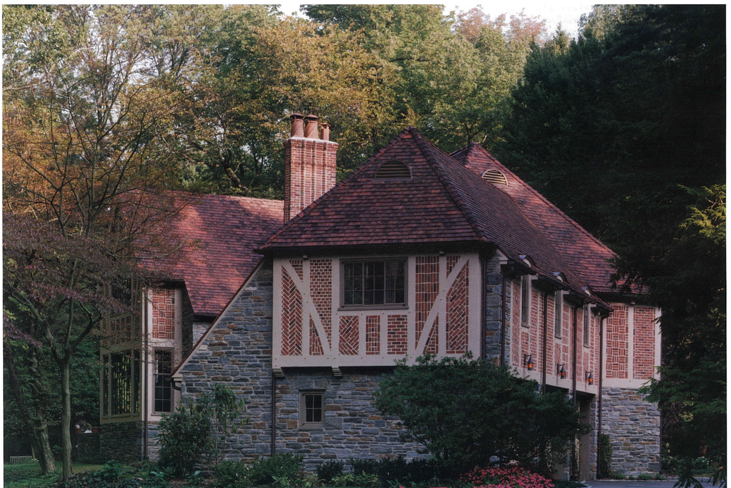
The oblique siting of the new garage hides the garage doors – by Artisan Custom Doorworks of Bristol, PA – from immediate view and opens the approach into the new entrance courtyard. The ironwood trees at the corner of the garage were protected during construction and give a sense of scale to the landscape; the azaleas were removed and replanted after construction.
