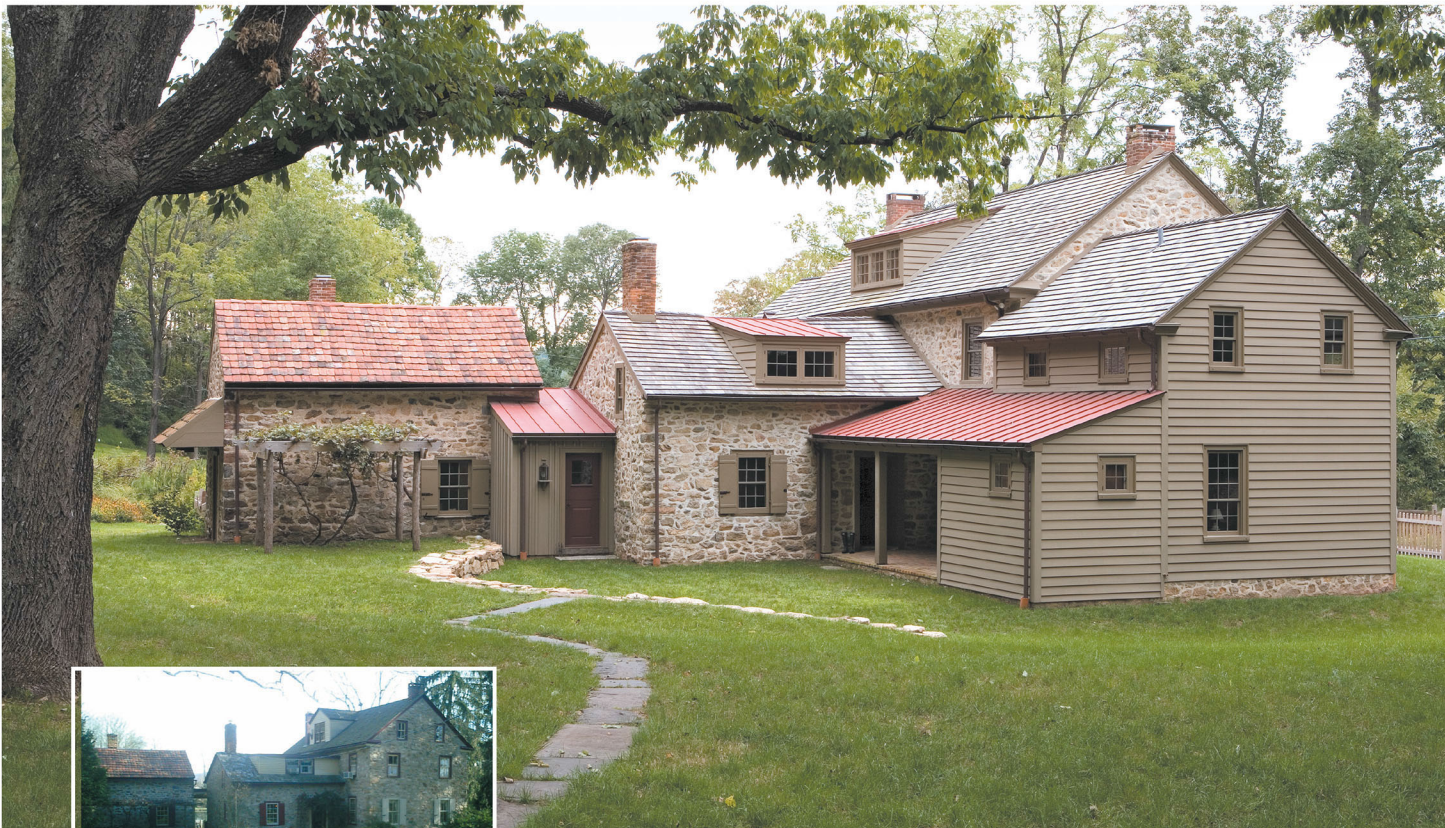
PZA connected the separation between the existing main house and the summer kitchen with the addition of a mudroom/potting room. The clapboard-sided library and rear porch were added to the west side of the house.
